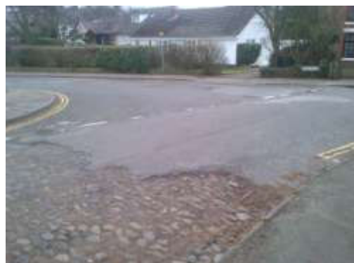
Intersection of old and new surfaces in Crown Bank and High Street. Poor intersection in crown Bank with loose edge of tarmac overlying cobbled street
