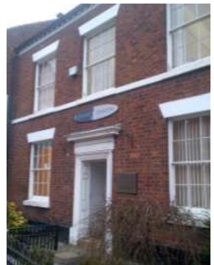
6 over 6 sash windows in this listed Georgian property. Also not the panelled door surround with pediment and dentil moulding to fascia board
