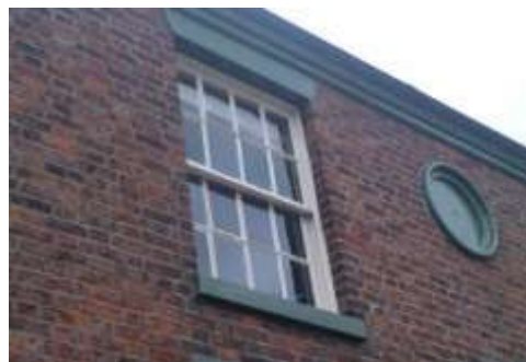
Flemish bond brickwork and 8 over 8 Georgian Sash window, High Street
